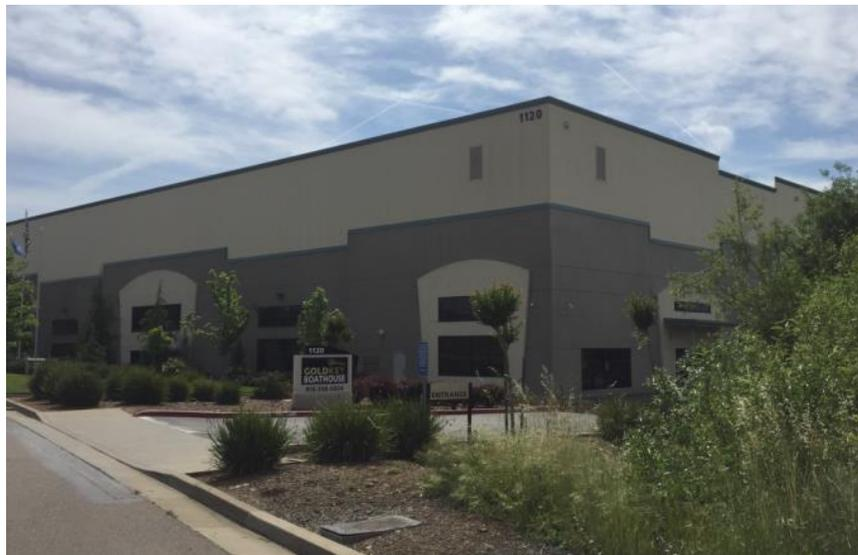
Tilt-up construction, as shown in this example, often have large expanses of open space where fires can spread, flashover is more intense, roof ventilation is required to remove smoke, and firefighters can easily lose their sense of direction in the smoke.
