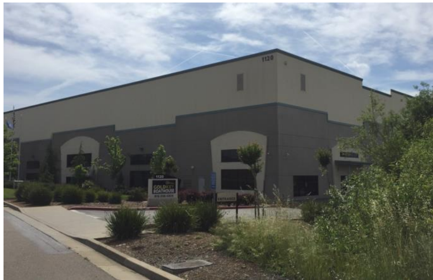
Figure 22—Tilt-up Construction
