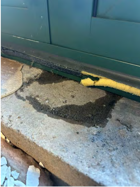
Image 7 – Water Present at Door Head
