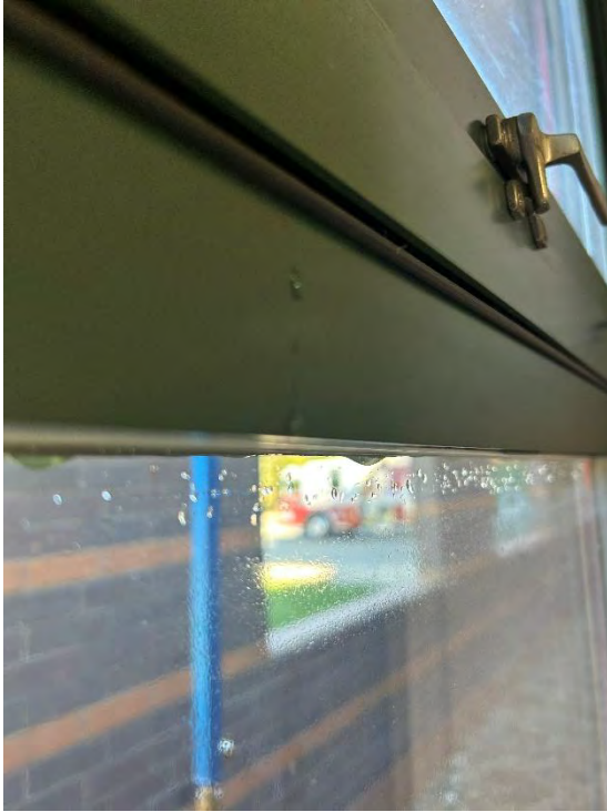
Image 9 – Window Glazing Failure
