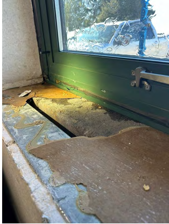
Image 8 – Glazing Failure at Door Bottom
