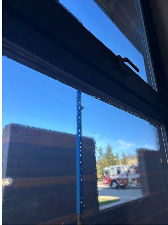
Image 10 – Window Glazing Failure
