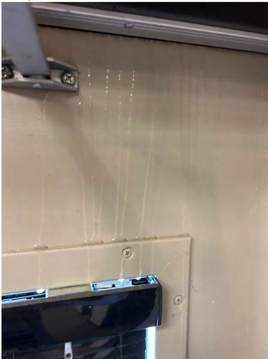
Image 7 – Water Present at Door Head
