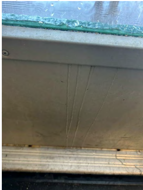
Image 8 – Glazing Failure at Door Bottom
